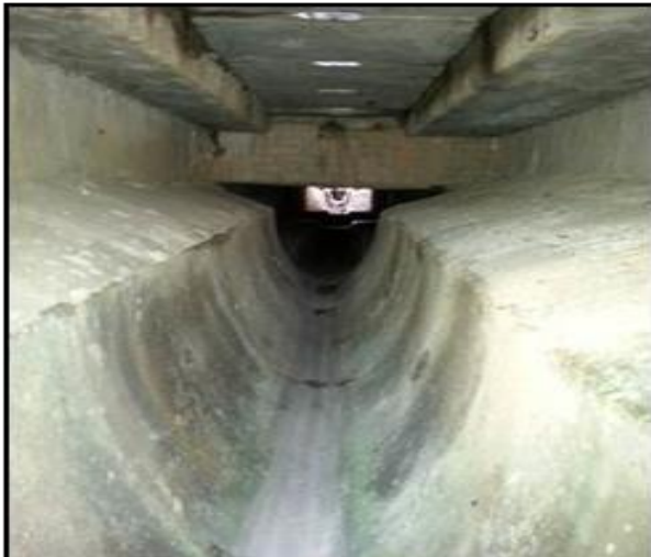
Smaller drains <2m width
