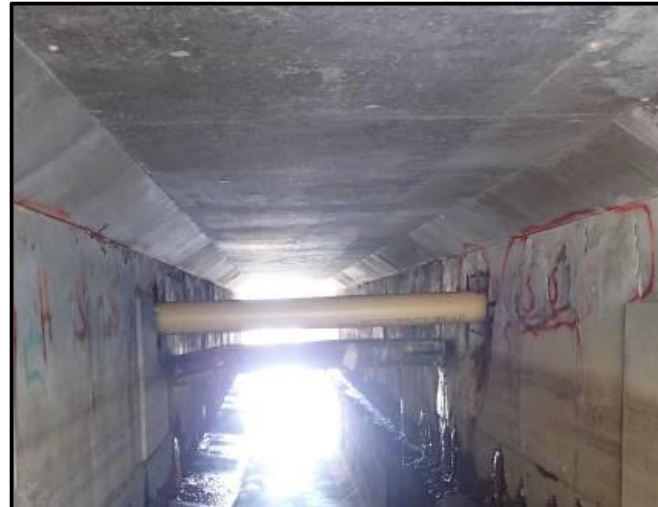
Services crossing drains
