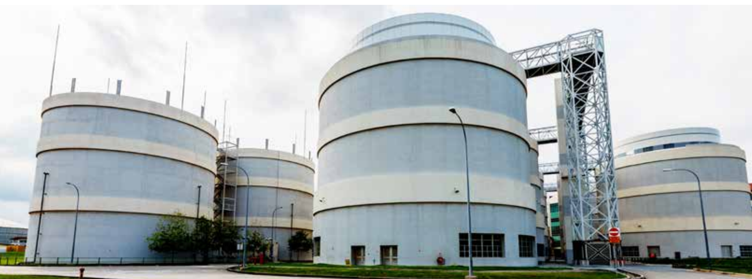
Anaerobic Digesters located at Changi Water Reclamation Plant, implemented under DTSS Phase 1.
