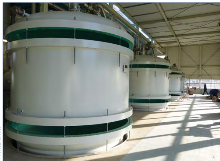
Fig. 1: The CeraMac® system developed by PWN Technologies uses a single stainless steel vessel to house up to 192 ceramic membrane modules
