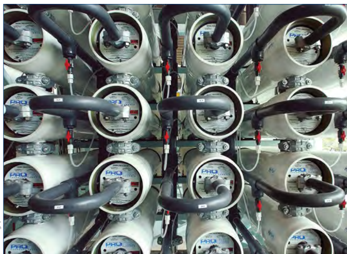
Fig. 1: Reverse osmosis is used to produce high-grade reclaimed water
