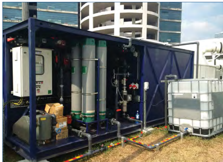
Fig . 2: Moving Bed Bioreactor technology with ultrafiltration membrane system at Ulu Pandan Water Reclamation Plant
