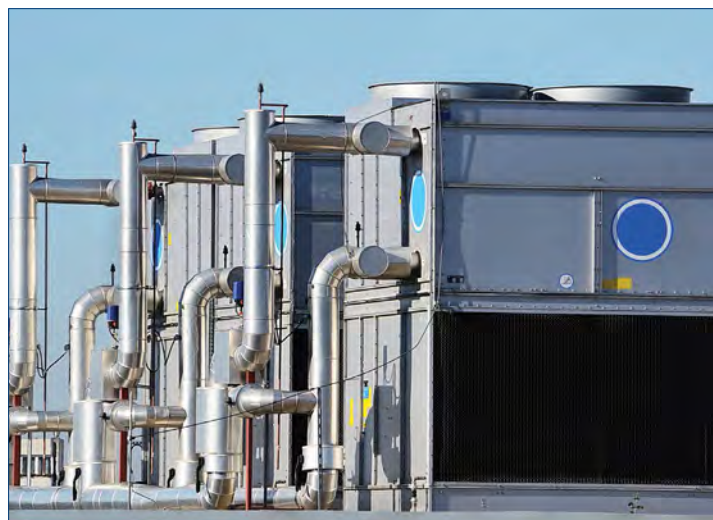
Fig. 1: Cooling towers that reject heat are an important component in the cooling systems of buildings
