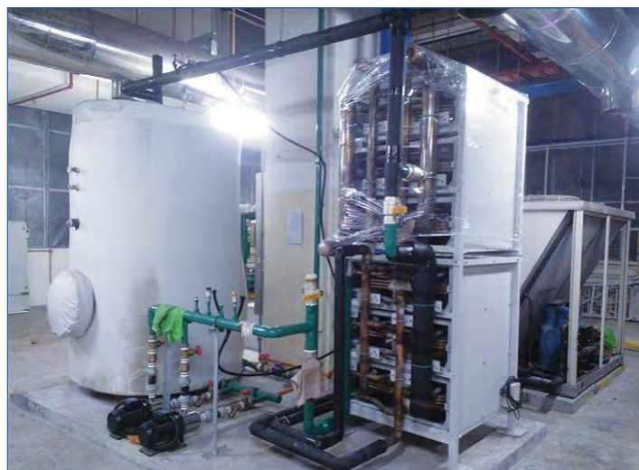
Fig. 2: Natflow's prototype heat exchanger developed and piloted at Changi General Hospital (CGH)
