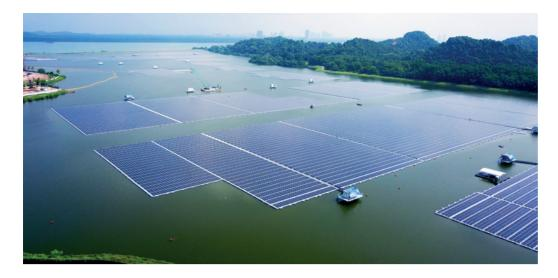
Figure 6. An aerial view of the Tengeh Floating Solar Farm which was launched in July 2021. This solar farm has a peak capacity of 60 megawatts, enough to power 16,000 four-room HDB flats for a year. Photo credit: Sembcorp Industries
