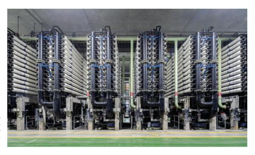
Figure 4. Direct coupling of the ultrafiltration process (on the right) with the downstream reverse osmosis process eliminates the need for intermediate break tanks and pumping, reducing energy and footprint. Photo credit: Keppel
