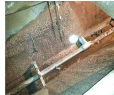
Primary Sludge Hopper with suction manifold
