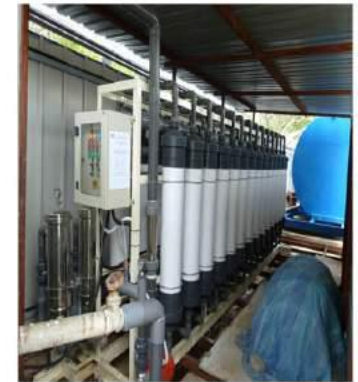
Membrane Ultrafiltration ECM Silt Treatment Plant from 5m 3 /hr. to 120m 3 /hr.
