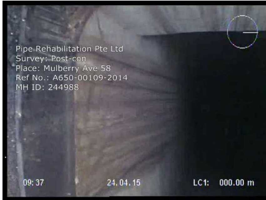
Photo: 244988-042415-M4.JPG General photograph, shaft wall (detail)
