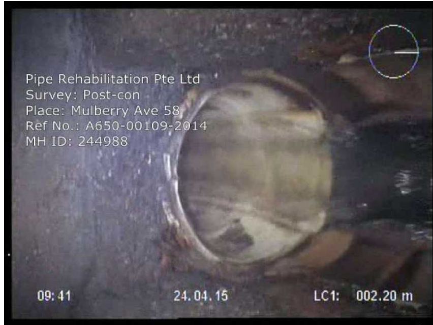
Photo: 244988-042415-M12.JPG General photograph, incoming pipe3
