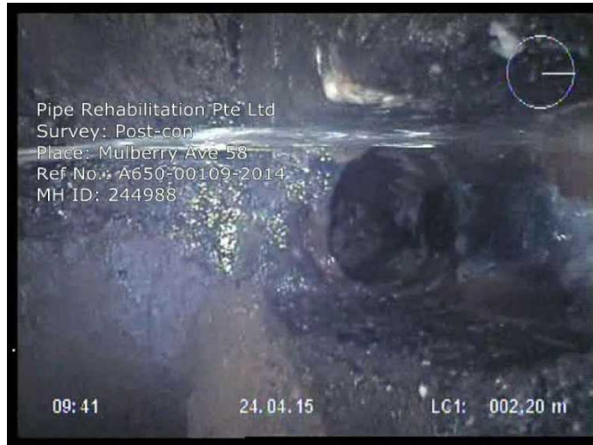
Photo: 244988-042415-M10.JPG General photograph, incoming pipe 1
