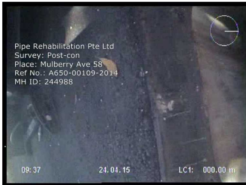
Photo: 244988-042415-M3.JPG General photograph, manhole frame (detail)
