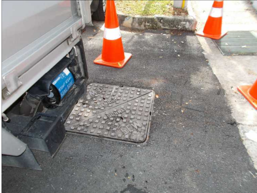
Photo: 244988-042415-M.JPG General photograph, manhole surrounding location
