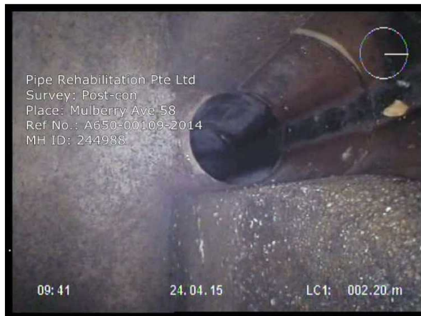
Photo: 244988-042415-M11.JPG General photograph, incoming pipe 2
