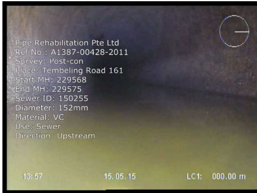
Photo: 150255-051515-S.jpg, 00:00:01 0m, Start of survey, upstream direction
