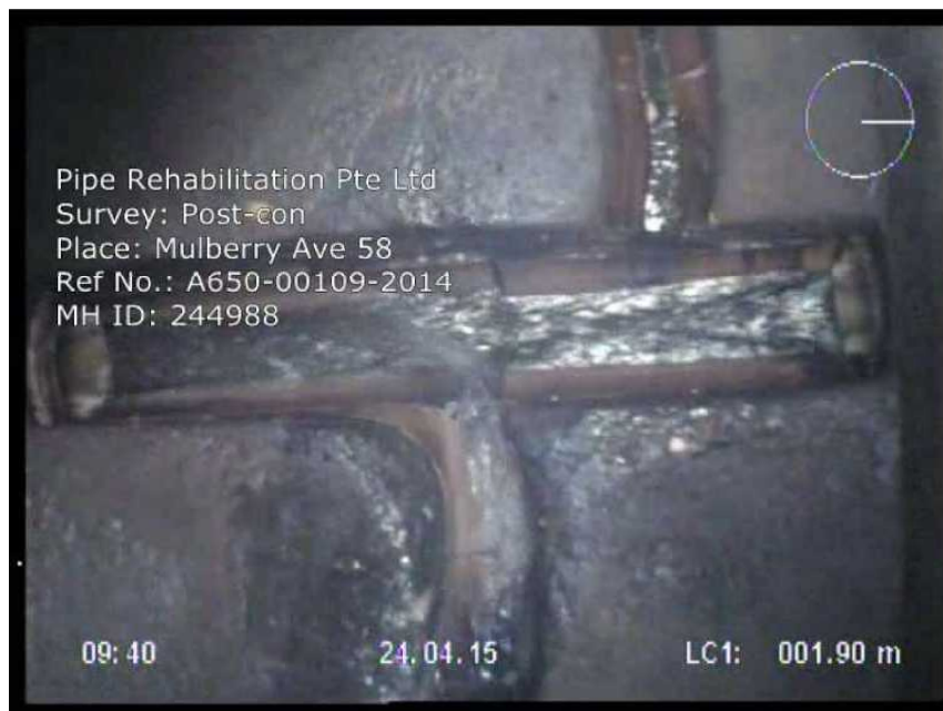
Photo: 244988-042415-M7.JPG General photograph, manhole benching
