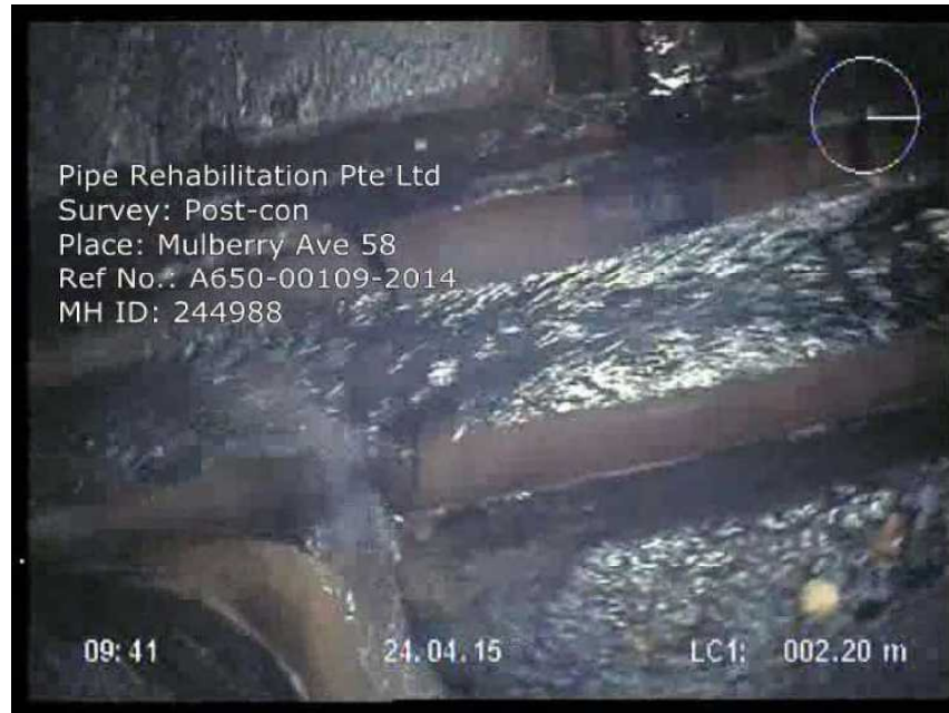
Photo: 244988-042415-M8.JPG General photograph, invert level
