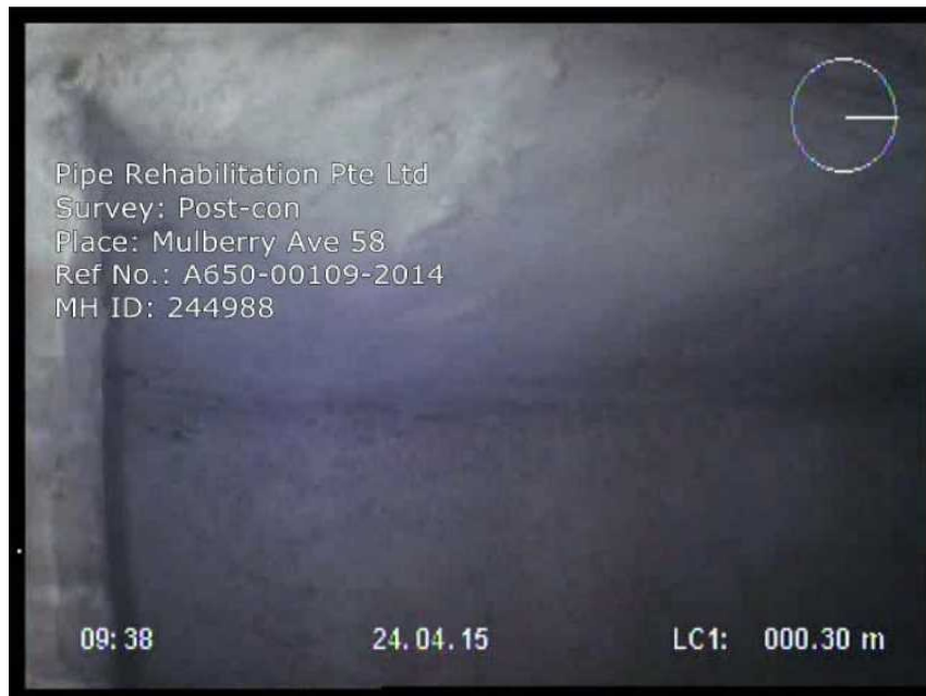
Photo: 244988-042415-M5.JPG General photograph, chamber wall
