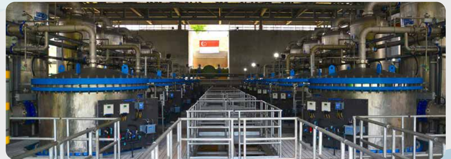
Ceramic membranes at CCKWW.
