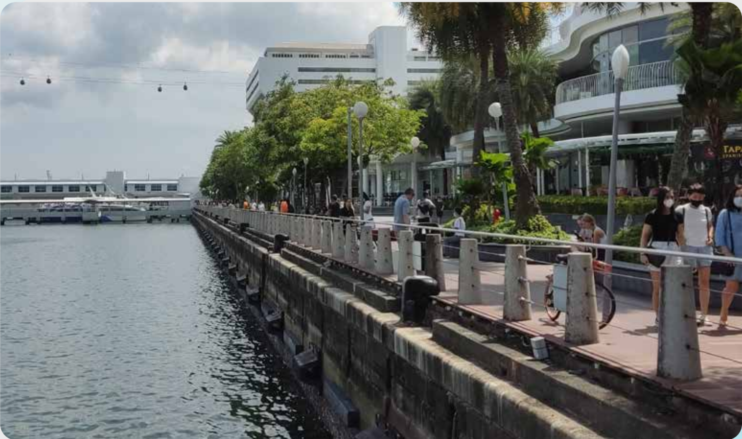
Possible coastal protection measures including hard engineering solutions such as seawalls designed to be multifunctional (for example, integrated with promenade) will be studied during the SSS.
