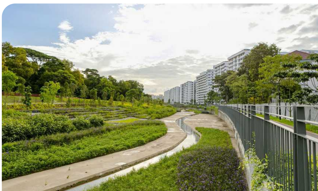
Figure 1.11 Acting as a pathway measure, Sungei Tampines is partially naturalised to integrate seamlessly with the adjacent Tampines Eco Green.
