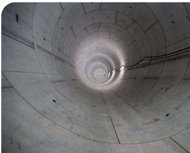
Figure 4.8 This 2km-long diversion canal runs underneath Tanglin Road to Grange Road, across to Hoot Kiam Road, off Kim Seng Road and to the Singapore River. This canal is 6m to 14m wide in diameter and located 3m to 4m below ground.
