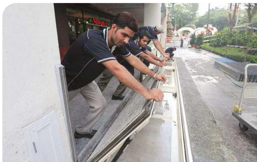
Figure 6.6 Regular tests and inspections of flood barrier systems are necessary to ensure that the system can be reliably activated during flood events.
