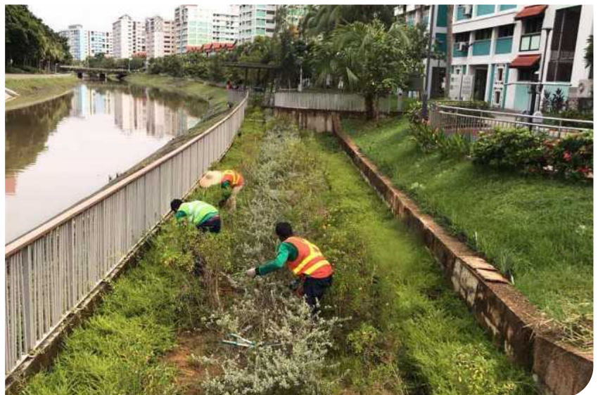
Figure 6.5 Sedimentation and excessive vegetation will grow inside the grass conveyance channel obstructing flow and reducing conveyance capacity during rain event. This could also potentially be a breeding ground for mosquitoes when stagnant water is trapped in bioretention feature. Regular maintenance is required to ensure its functionality.
