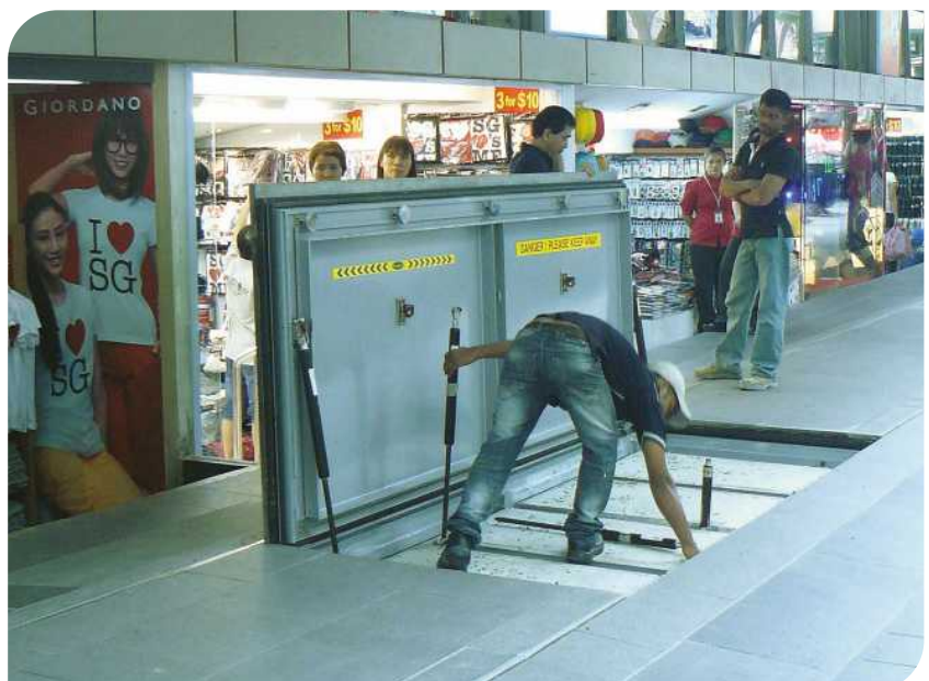
Figure 5.12 Maintenance staff checking and testing a flip-up flood barrier.
