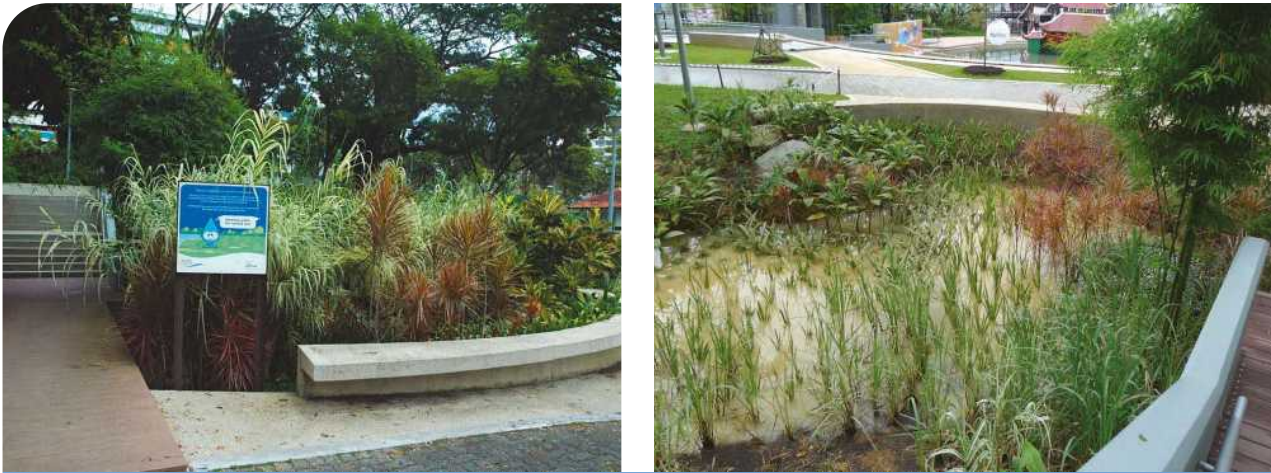
Figure 6.3 A low seat wall, together with clear signage, can be used to limit access into the bioretention feature.
