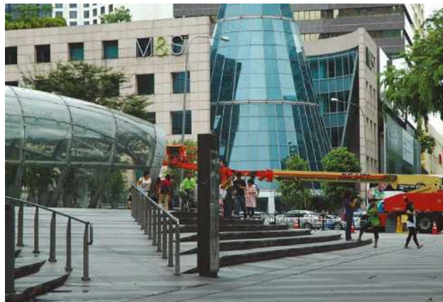
Figure 5.3 Steps and ramps are some of options to achieve the minimum platform levels for developments with entrances to underground facilities.
