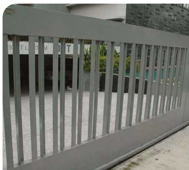
Figure 5.16 The entrance gate of this development leading directly to the basement car park was designed with a solid bottom section, with openings (for aesthetics) starting at the level above the required minimum crest level. A cross-section schematic of the gate is shown on the right.
