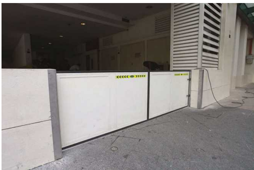
Figure 5.24 Swing-type flood barrier in open (top) and closed (bottom) positions at access to loading/unloading areas.
