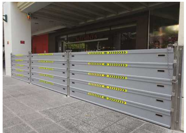
Figure 5.23 A multi-slot barrier at the front of Tanglin Mall before (left) and after (right) installation. These barriers have to be installed manually.
