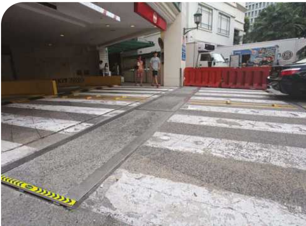
Figure 5.22 A flip-up barrier at the entrance to the basement carpark in closed (left) and open (right) positions.
