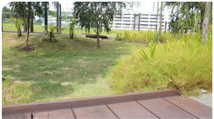
Figure 6.4 Erosion in grass swales can be minimised by planting more resilient or water-tolerant species in areas that experience higher flow velocities or are frequently submerged (e.g. depression areas).
