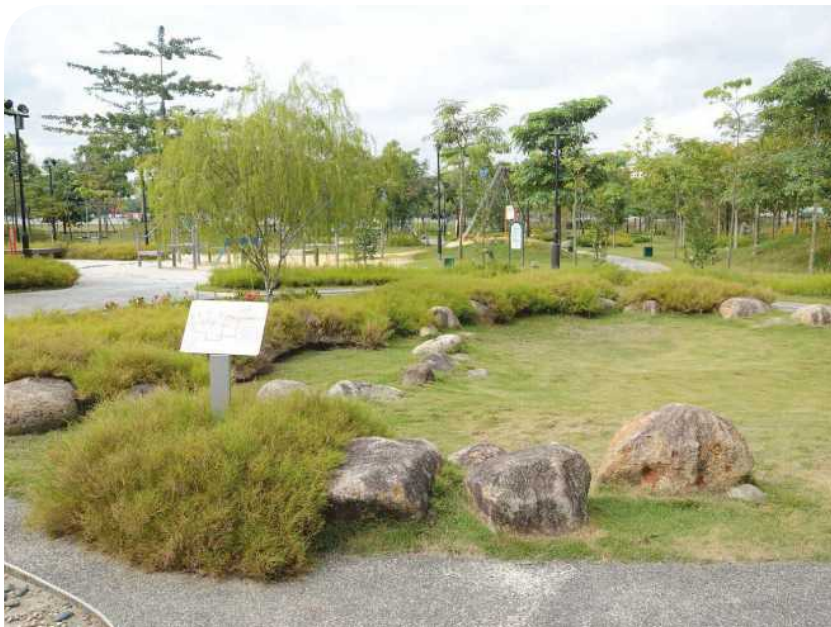
Figure 6.2 Using a combination of gradual slopes and clear signage, this dry pond allows users to move out of the area safely and easily during a rain event.
