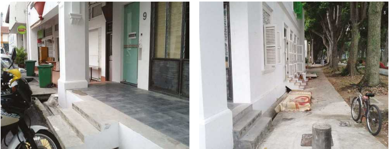
Figure 5.7 For this corner unit shophouse, the five-foot way was raised to match entrance levels. Steps were created to lead down to the road and common sidewalk area for the side entrances.
