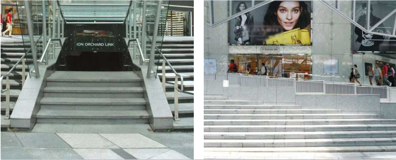
Figure 5.4 Additional crest protection levels are required for developments with underground linkages to MRT stations (e.g. Ion Orchard Link) and for all openings to basement facilities, including ventilation ducts (e.g. Wisma Atria)
