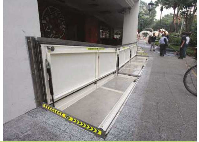
Figure 5.21 Flip-up barrier at the front of Tanglin Mall, in closed (left) and open (right) positions. This barrier was chosen to achieve seamless connectivity for pedestrians crossing the junction of Tanglin and Grange Road to Tanglin Mall.
