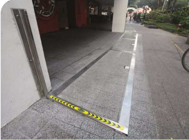
Figure 5.21 Flip-up barrier at the front of Tanglin Mall, in closed (left) and open (right) positions. This barrier was chosen to achieve seamless connectivity for pedestrians crossing the junction of Tanglin and Grange Road to Tanglin Mall.
