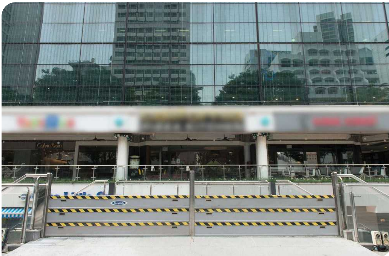
Figure 5.17 Slot-in flood barriers.
