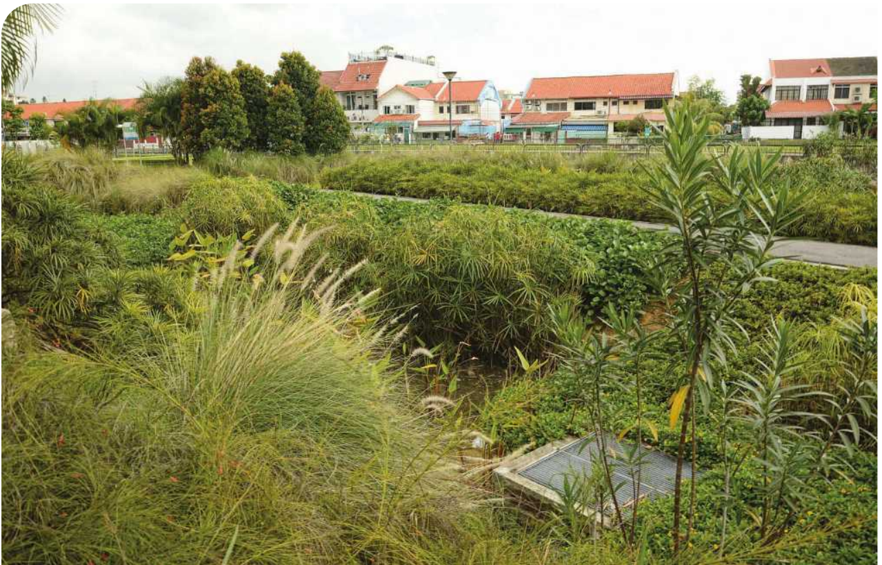
Figure 3.15 A bioretention basin at Balam Estate with an overflow pit.
