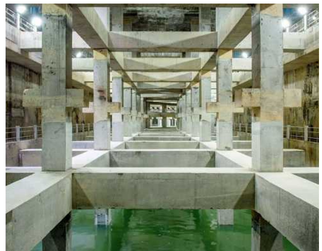
Figure 4.9 The SDT can hold up to 38,000m 3 or 15 Olympic sized swimming pools of stormwater which can be emptied in four hours to prepare the tank for the next heavy rainfall.
