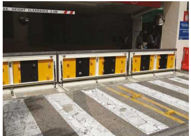
Figure 5.22 A flip-up barrier at the entrance to the basement carpark in closed (left) and open (right) positions.
