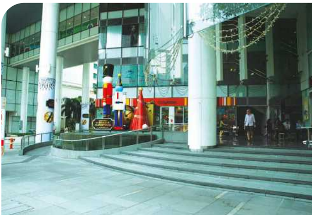
Figure 5.3 Steps and ramps are some of options to achieve the minimum platform levels for developments with entrances to underground facilities.
