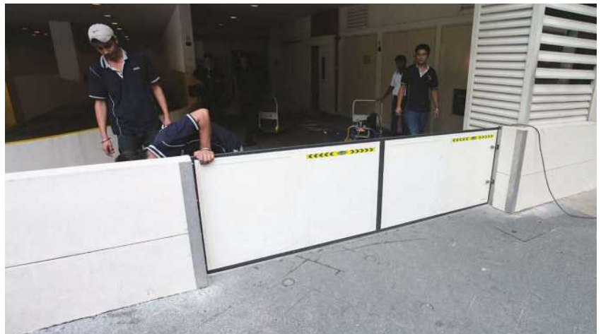
Figure 5.14 Manually operated swing-type barrier system.
