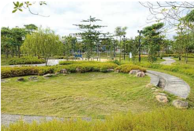
Figure 3.14 Dry pond at Greenwood Sanctuary - During rain events, stormwater runoff flows from the surrounding ground to the dry pond and filters to underground percolation tanks encased in a permeable membrane layer. During dry weather, the lawn area in the dry pond can also be used for recreational activities.
