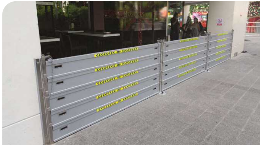
Figure 5.13 Manually installed slot-in barrier system.
