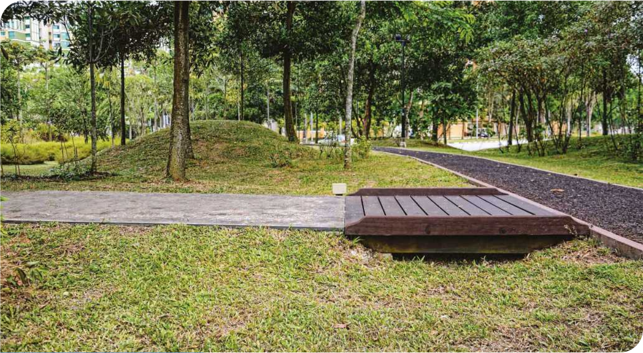
Figure 6.1 A crossing installed across a grass conveyance swale ensures a smooth transition between the two walkways, and also protects the soil beneath from being compacted by pedestrians, which would otherwise reduce the infiltration capacity of the swale.
