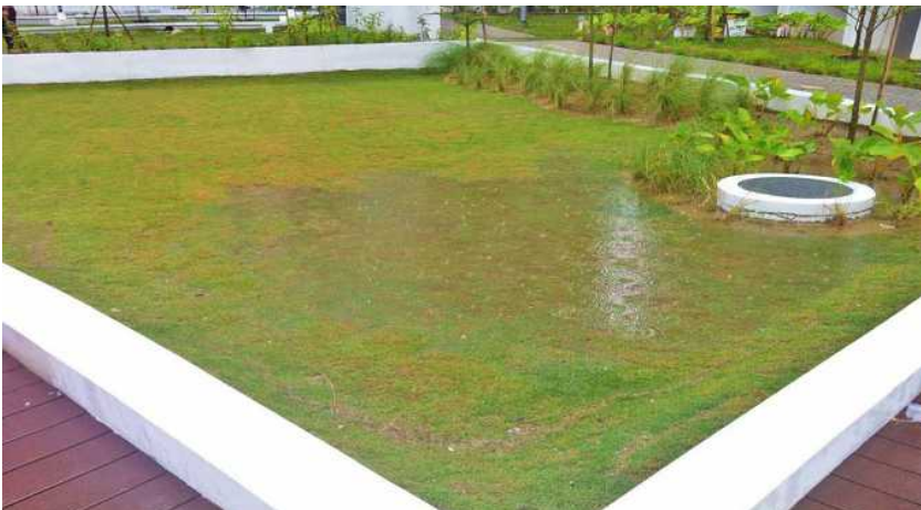
Figure 3.25 Bioretention basin serving as a multi-purpose lawn during dry weather. During a rain event, it temporary stores stormwater runoff. (Images courtesy of Henning Larsen)
