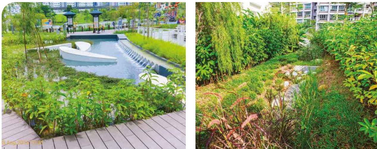
Figure 3.22 Bioretention basin during dry weather (left). During a rain event (right), stormwater is directed into the swale, reducing the velocity and volume of runoff into the drainage system.
