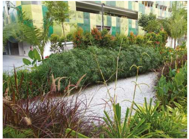
Figure 3.19 Example of a gravel trench serving as a conveyance channel for stormwater runoff.
