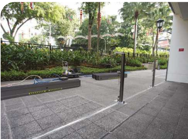
Figure 5.23 A multi-slot barrier at the front of Tanglin Mall before (left) and after (right) installation. These barriers have to be installed manually.
