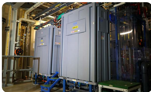
Micron's EDR technology utilises less space than conventional treatment processes.
