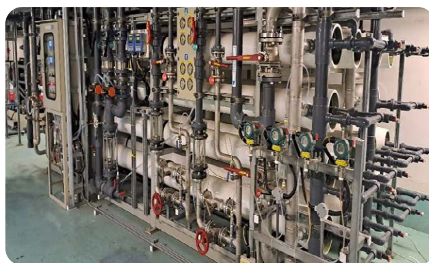
UMC's diluted HF system recycles process wastewater for secondary facility system usage.
