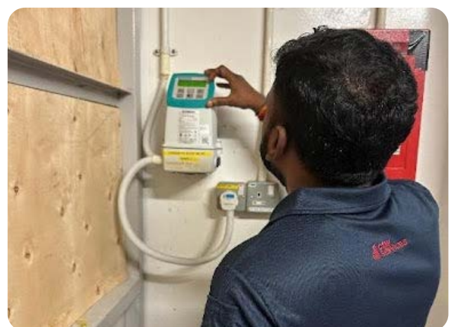
The Metropolis uses meters to track the amount of air conditioning condensate water recycled.
