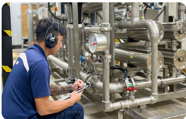
AML's reverse osmosis system diverts reject water back to water tanks for reuse.
