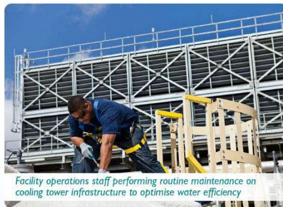
Google's custom-engineered cooling systems, built to maximise water efficiency
