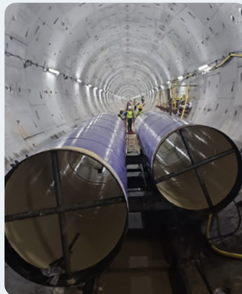
1.2-metre-diameter NEWater pipe laying inside the completed 6-metre-diameter tunnel.
