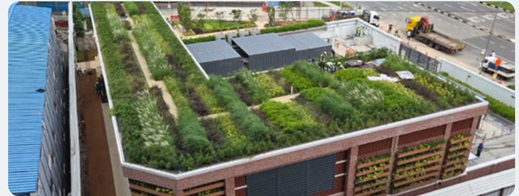
Syed Alwi Pumping Station.
