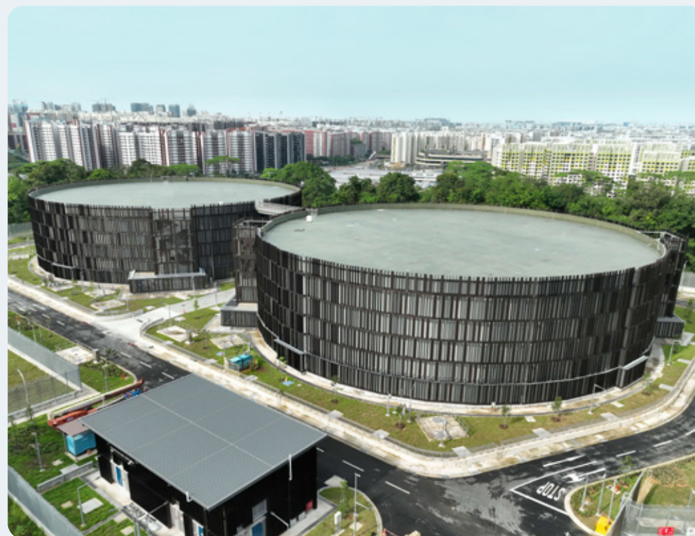
Aerial shot of Tengah Service Reservoir at Bukit Batok Road.
