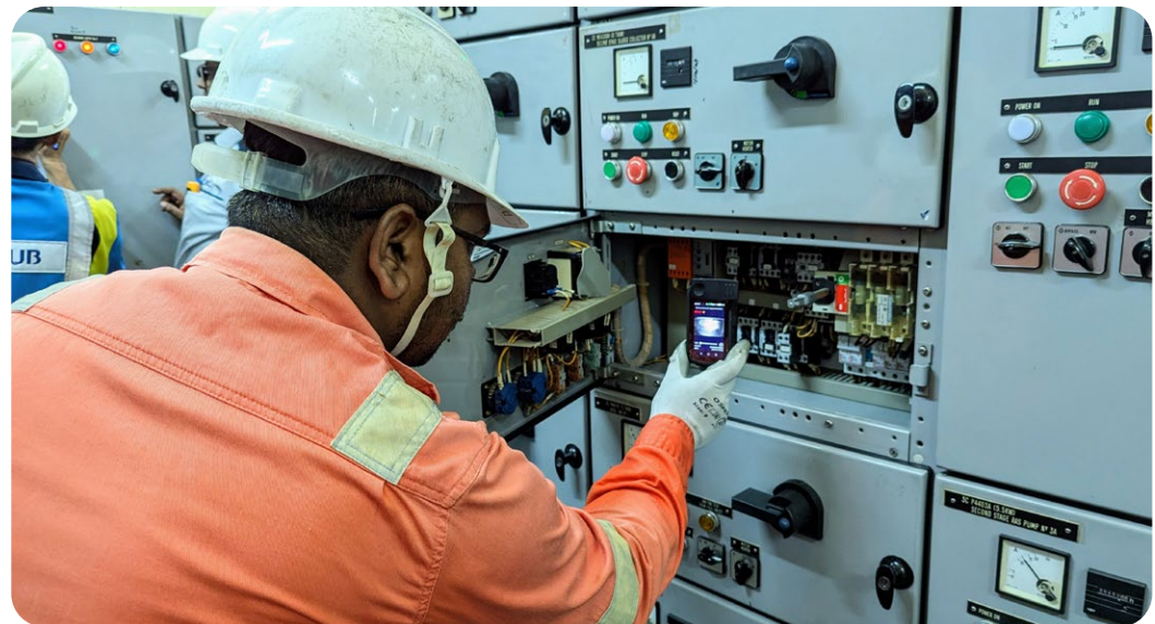
Worker using the PUB Enterprise Wearables System to livestream their work for real-time support.
