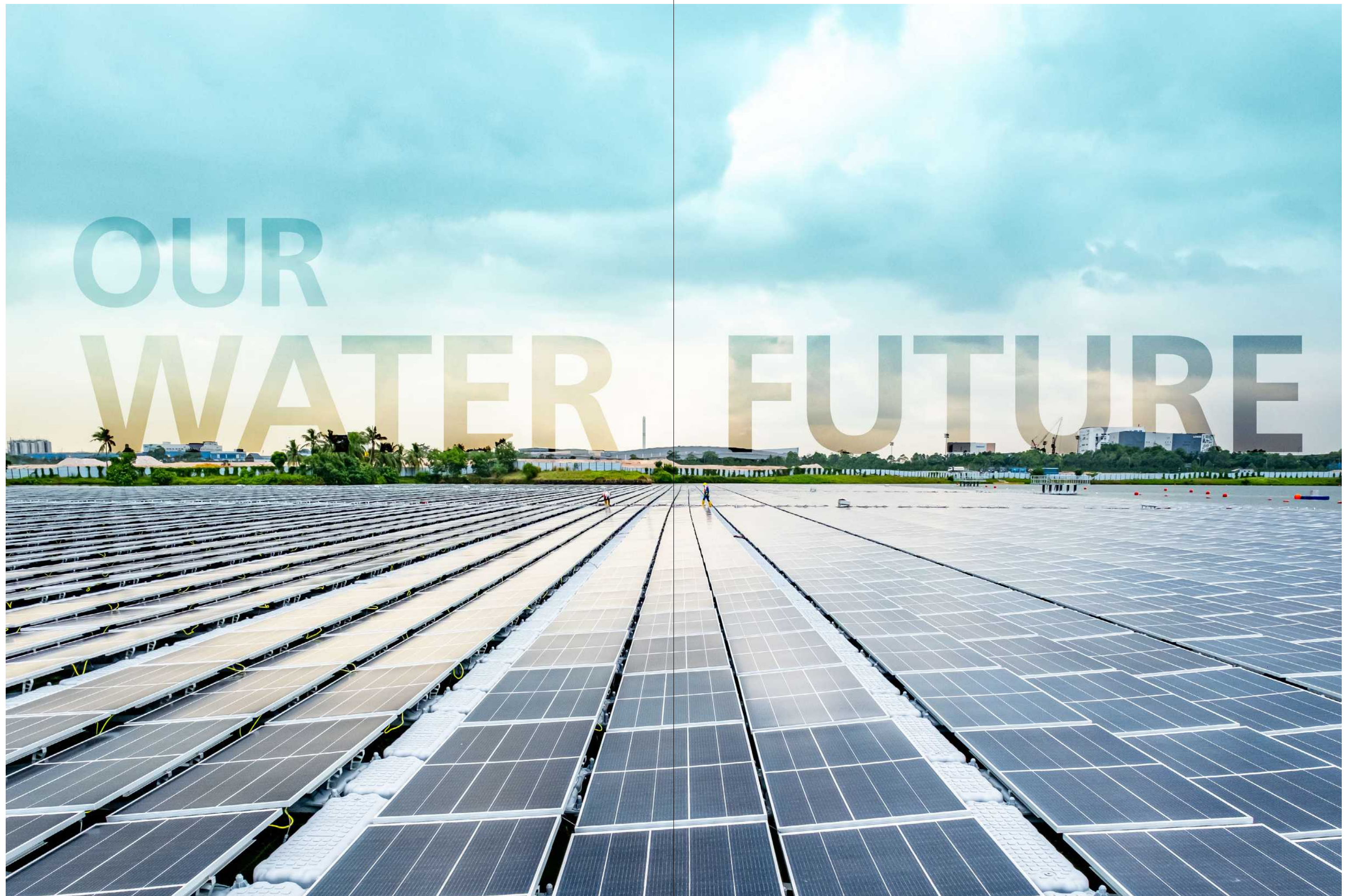
The 60 MWp floating solar farm on Tengeh Reservoir is one of the world's largest inland floating solar farms, comprising 122,000 solar panels over 38 hectares.
