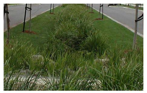
Figure 6.13 Photograph of bioretention swale
