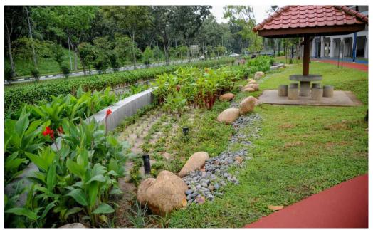
Figure 7.1 Example of bioretention basin in Sungei Tampines
