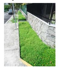
Figure 5.4 Swale incorporated into road reserve
