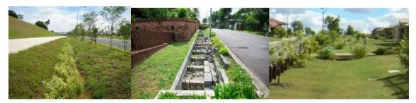
Figure 5.3 Swale systems: heavily vegetated (left), use of check dams (centre), grass swale with elevated crossings (right)
