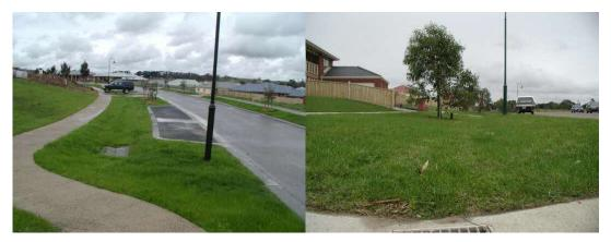
Figure 5.15 Similar buffer swale system for conveying runoff
