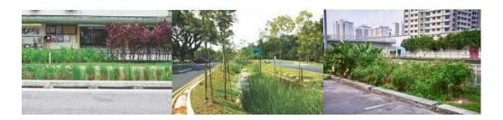
Figure 6.9 Kerb Arrangements with Breaks to Distribute Inflows on to Bioretention Swales and Prevent Vehicle Access
