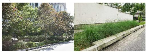
Figure 5.10 Kerb arrangements to promote distributed flow into swales
