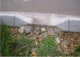
Figure 7.11 Typical Inlet Scour Protection Detail for Bioretention Basins Receiving Piped Flows
