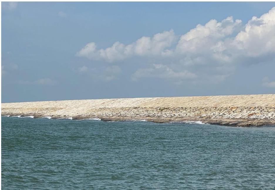
The natural rock layer covering the seaward side of the coastal dike's wall sensitively integrates the polder's coastline with its natural surroundings. (Credit: HDB)
