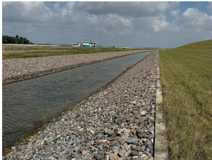
The seepage drain on the landward side of the coastal dike (Credit: HDB)
