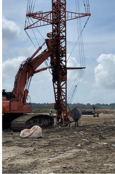
PVDs were inserted to drain water out of the clayey soil. (Credits: HDB)
