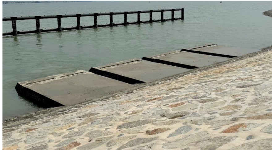
Multiple outlet structures run through the coastal dike and help channel excess water from the polder out into the sea. (Credit: HDB)
