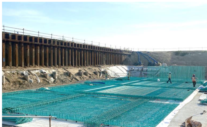
Cofferdams installed to keep construction areas dry. (Credit: HDB)
