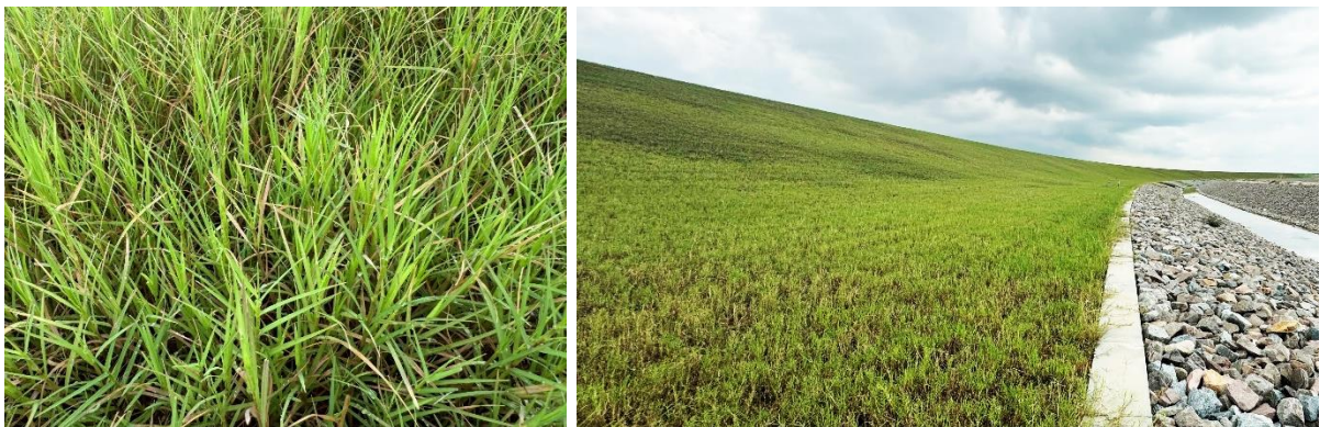
Bermuda grass (left) covers the landward side of the coastal dike (right) to mitigate erosion, while beautifying the landscape. (Credit: HDB)
