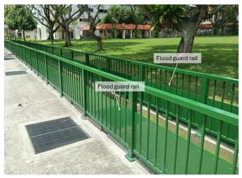
**Downstream measure:** Flood boards were mounted onto drain railings to prevent overspill of stormwater from the drain onto adjacent land.
