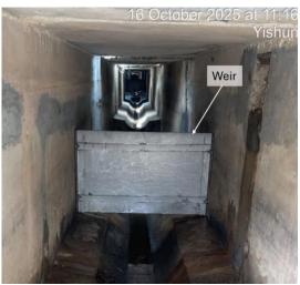
**Upstream measure:** Weirs were installed to slow down stormwater flow into downstream roadside drains.
