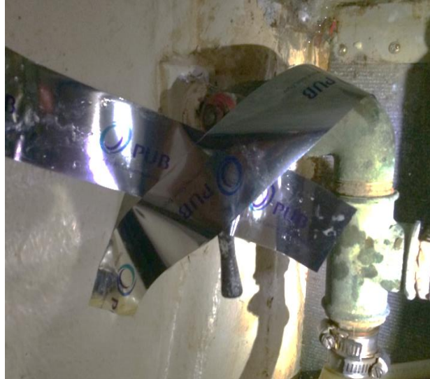
Photo of PUB secondary seal over a 'Y' valve
