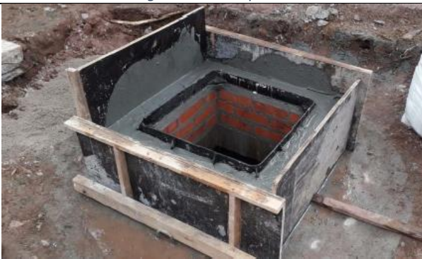
Figure 8: Casting of new engineering brickwork
