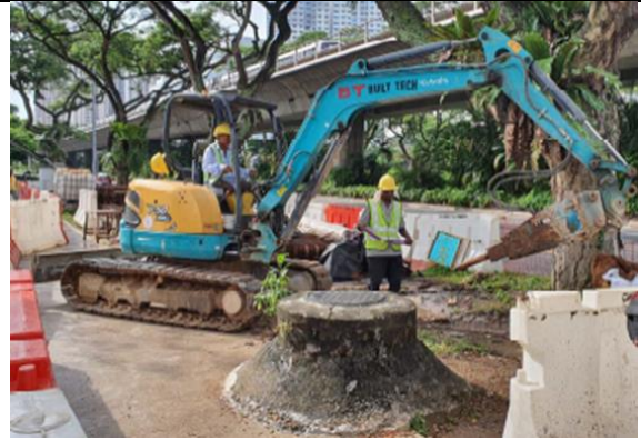
Figure 3: Existing Manhole condition (Close view)
