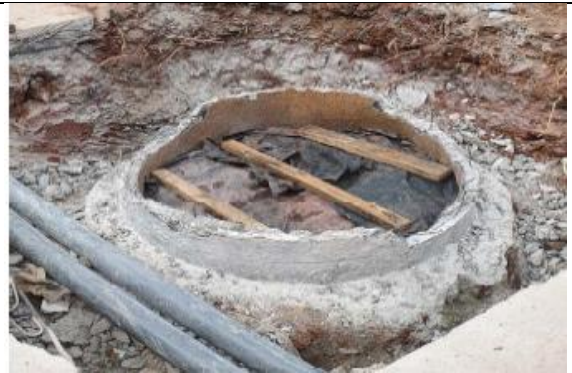
Figure 5: Breaking existing chambers - If applicable
