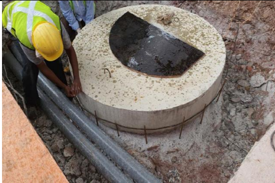
Figure 6: New top slab
