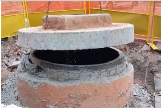
Figure 4: Removal of top slab - If applicable
