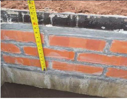
Figure 9: New brickwork measurement
