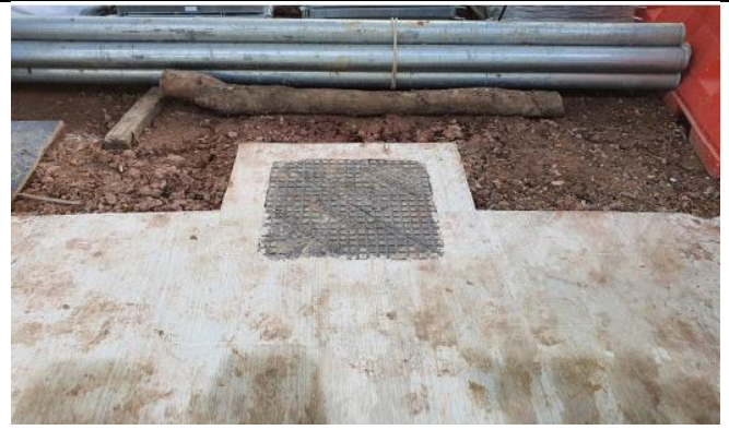
Figure 10: Manhole site condition (Close view)
