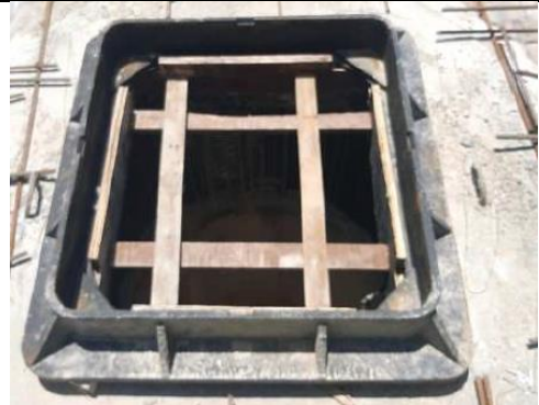
Figure 7: Heavy or medium duty cover installed
