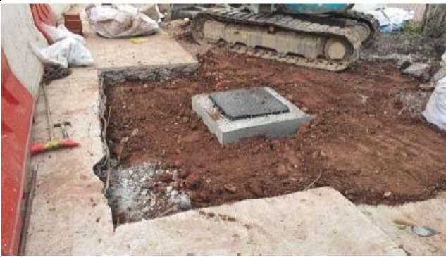
Figure 11: Manhole site condition (Far view)
