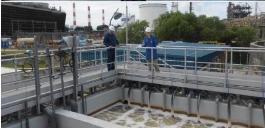
Churman's visit to a petrochemical complex (top) and a submerged ceramic membrane system treating refinery wastewater on Jurong Island (bottom).
