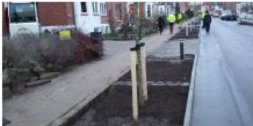
Ongoing roadbed projects in Skibhus area.
