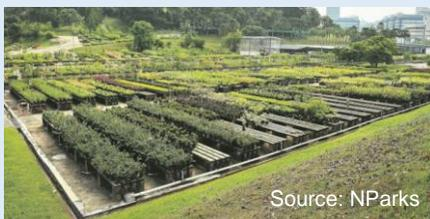
Cut-off drain channels rainwater runoff to the water treatment pond and pond water can be used for irrigation
