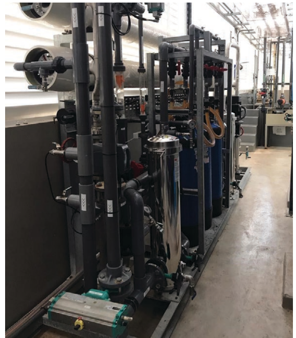
Figure 11: Waste Water Reclamation System
