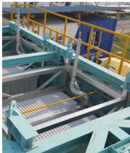
Fig. 2: Installation of the LENA MBR pilot plant
