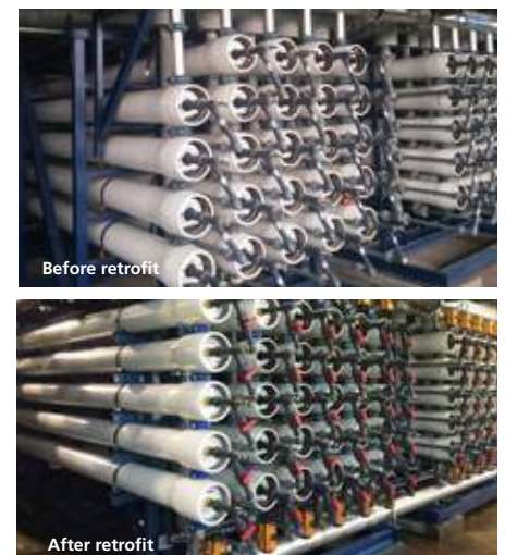
Fig. 2: Retrofitting project at Kranji NEWater Factory
