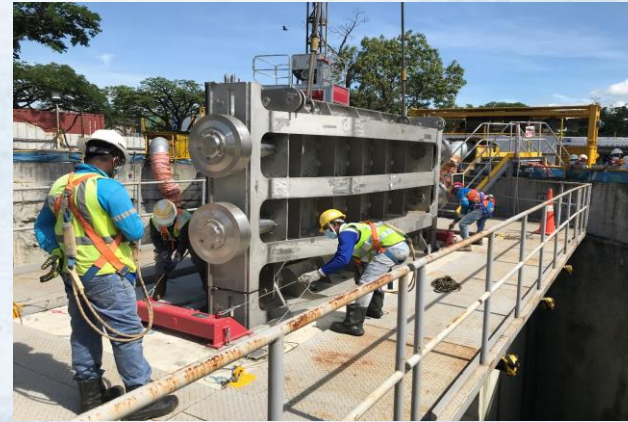
Assembly of the gate module in Dec 2020
