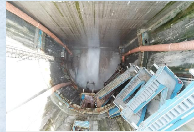
Lifting of roller gate in Dec 2020
